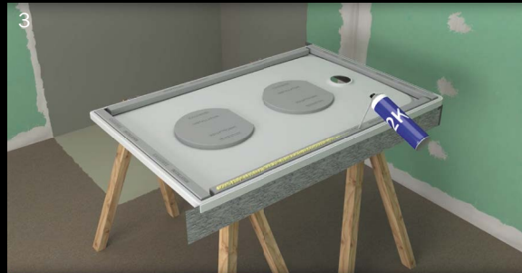
3 Add low expansion foam adhesive on pre-assembled tray support
