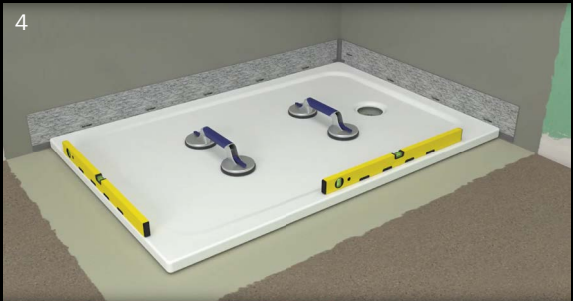
4 Turn shower surface with tray support over and place on floor, install drain fitting. Seal shower area – perfect with KALDEWEI Flex sealing set.
