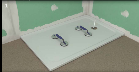
1 Align shower area and draw in drain position
