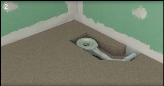
2 Create floor recess (screed, wooden floors) and connect drain fitting
