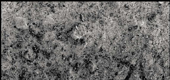
Grout in the tiled area rough, porous
